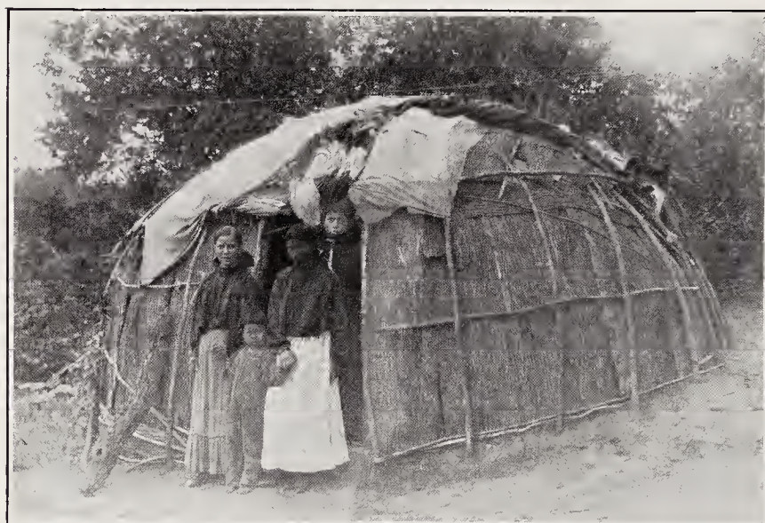
b. LODGE MADE OF BARK WITH COVERING OF REED MATTING
